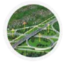
○ Long Dau Giay - Phan Thiet Expressway
